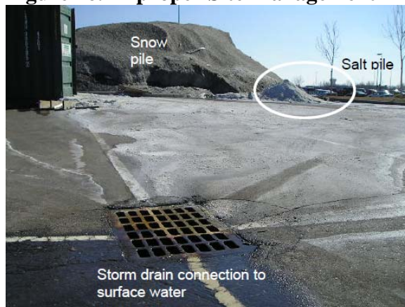
Figure 26. Improper Site Management
